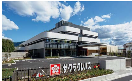
SAKURA Osaka Factory
